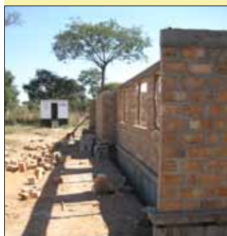
Two-classroom block under construction
