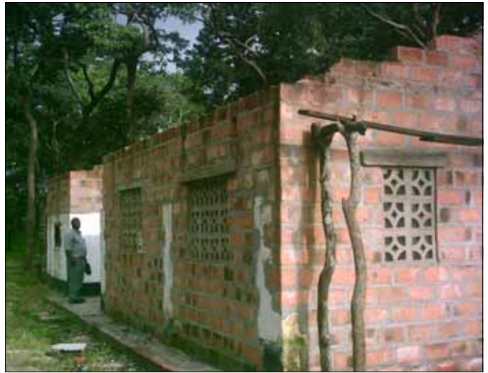
LBCS building refurbishment moves forward
